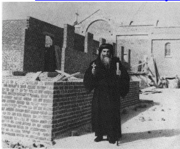
THE BUILDING OF ST. MINA'S MONASTERY
